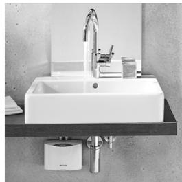
4 Unvented installation (closed outlet) with tap for pressurised appliances
